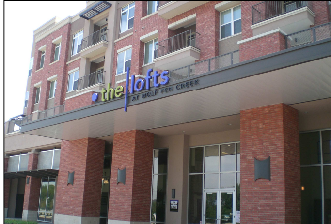
Figure 1 – Example of awning at building entrance
