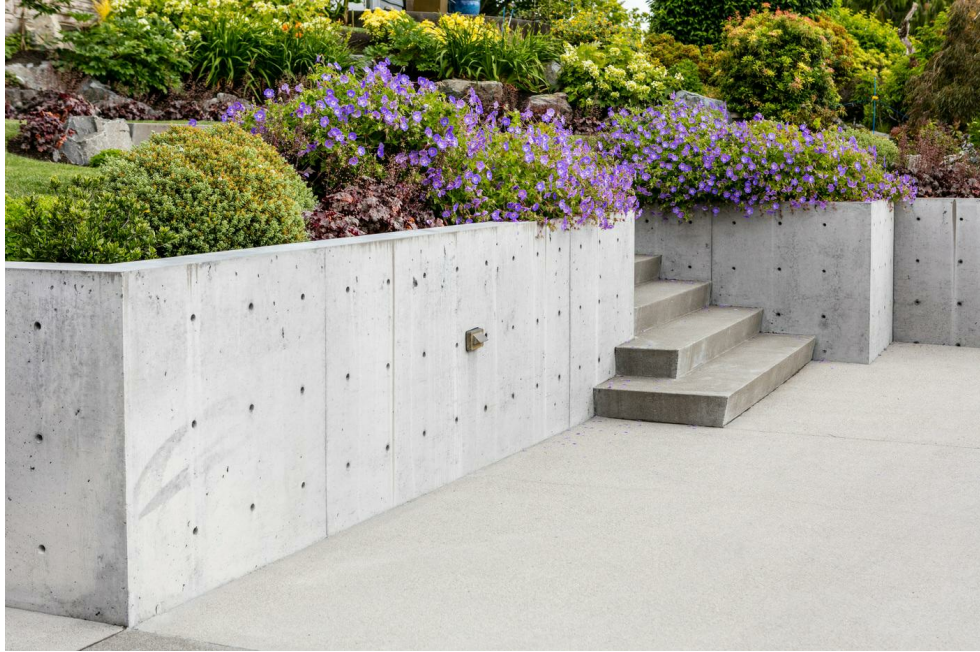
CONCRETE WALL - ARCHITECTURE FINISH
